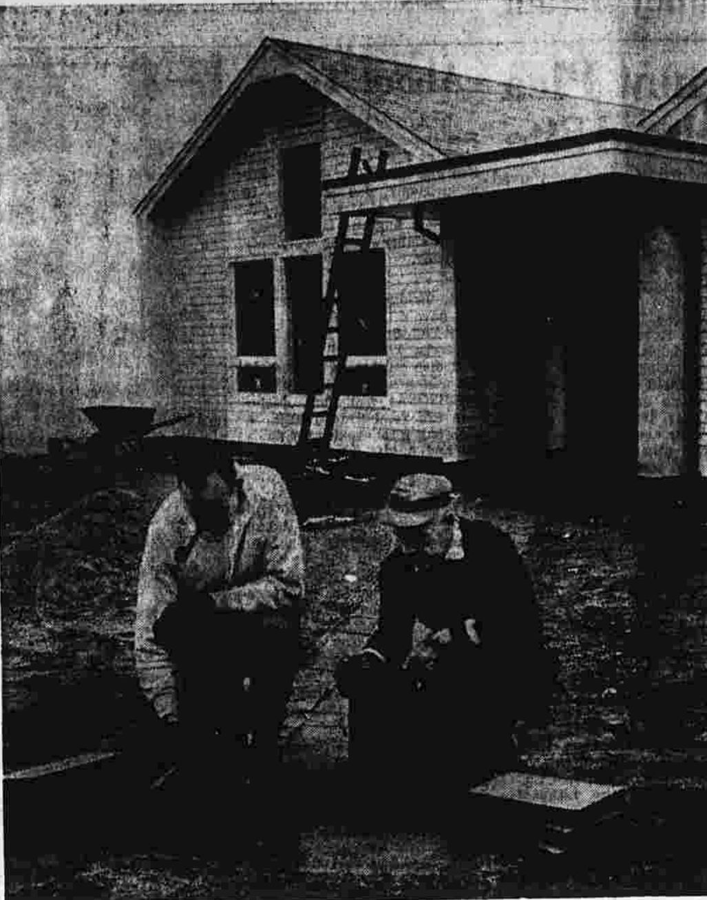
Parishioners Howard Horsman, left, and John Elliott laying tile for walk.
